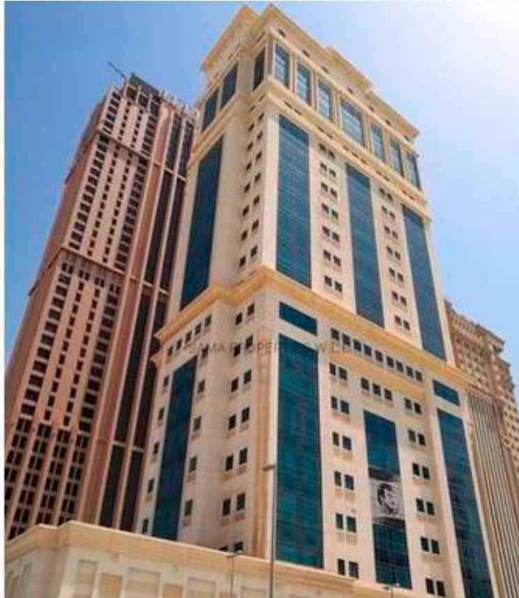
MEP works & AMC at Al Zubeira tower, West Bay
